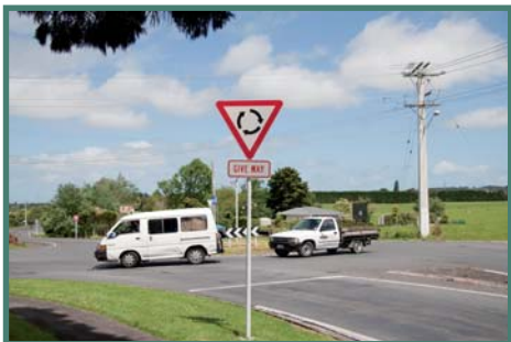
Mill Road roundabout.
