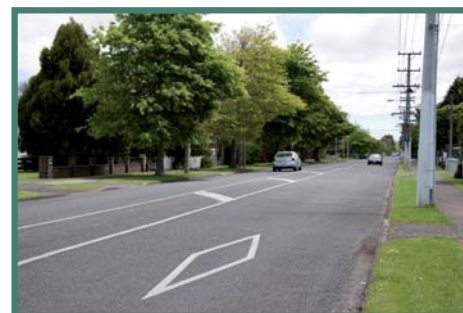
Cosgrave Rd looking north.
